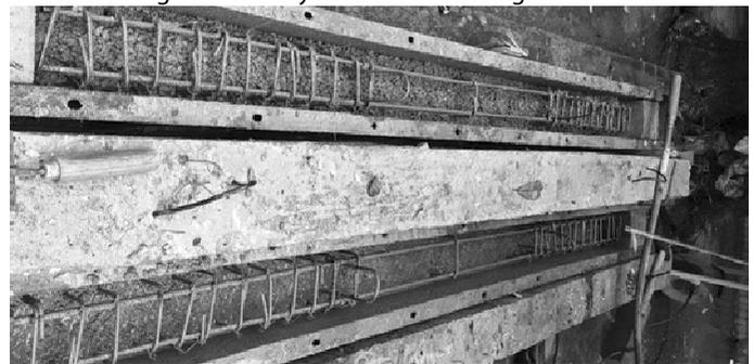
**Fig. 3** Concreting beams in layers
